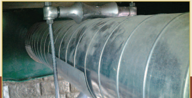
The Rovanco product does not require any special guides or saddles. This picture shows the piping installed under a bridge.
